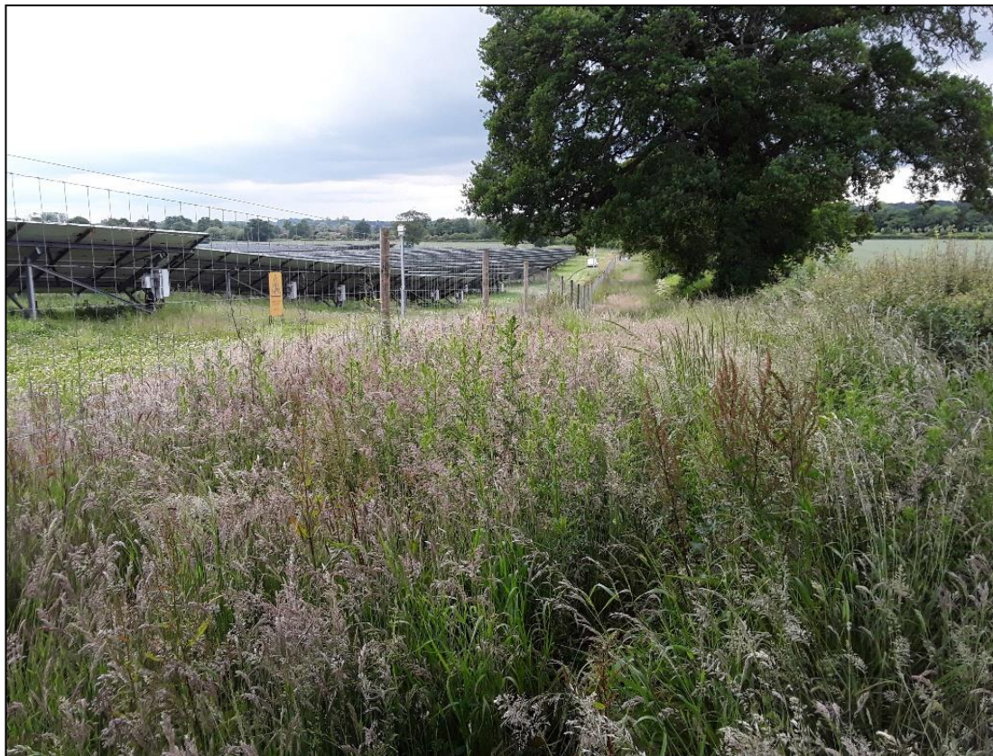
Figure 5: Tussocky Field Margin Created Between Security Fencing and Field Boundary
